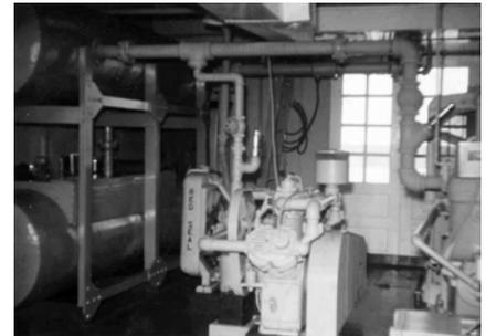
The compressor and air tanks to operate the foghorns.
